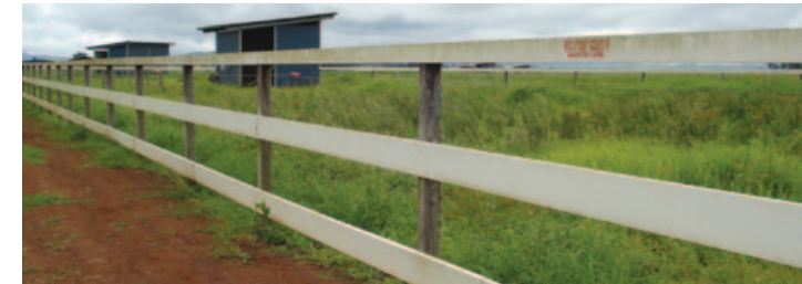
Post and rail fences can be made from wood or plastic. This one is also electric.
